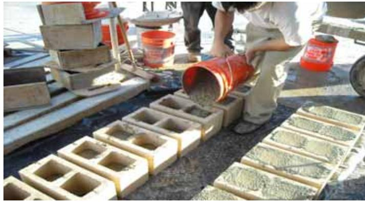
**Figure 1: Grout Placement in Concrete Masonry Unit Cells**
