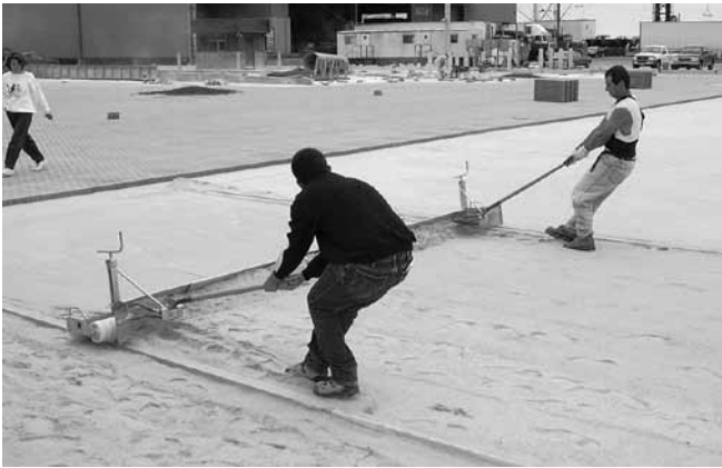
Figure 4. A two-man hand pulled screed
