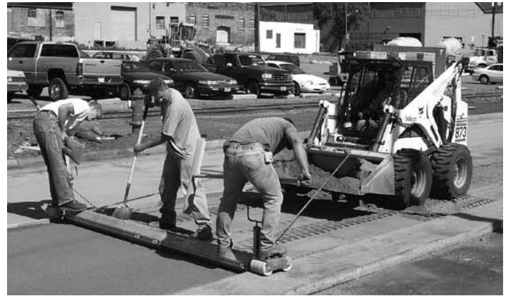
Figure 5. Mechanical screeding is the most efficient method of bedding sand installation
